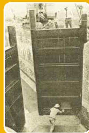
Restoring the gate for Lock 22 in Devizes, 1990
